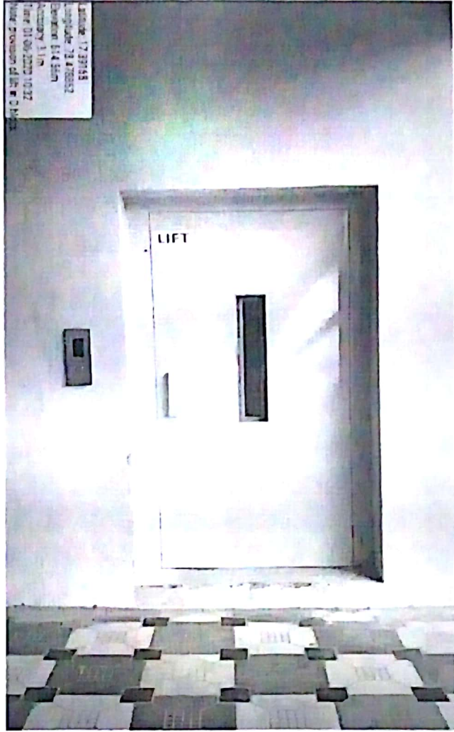
LIFT IN D BLOCK
