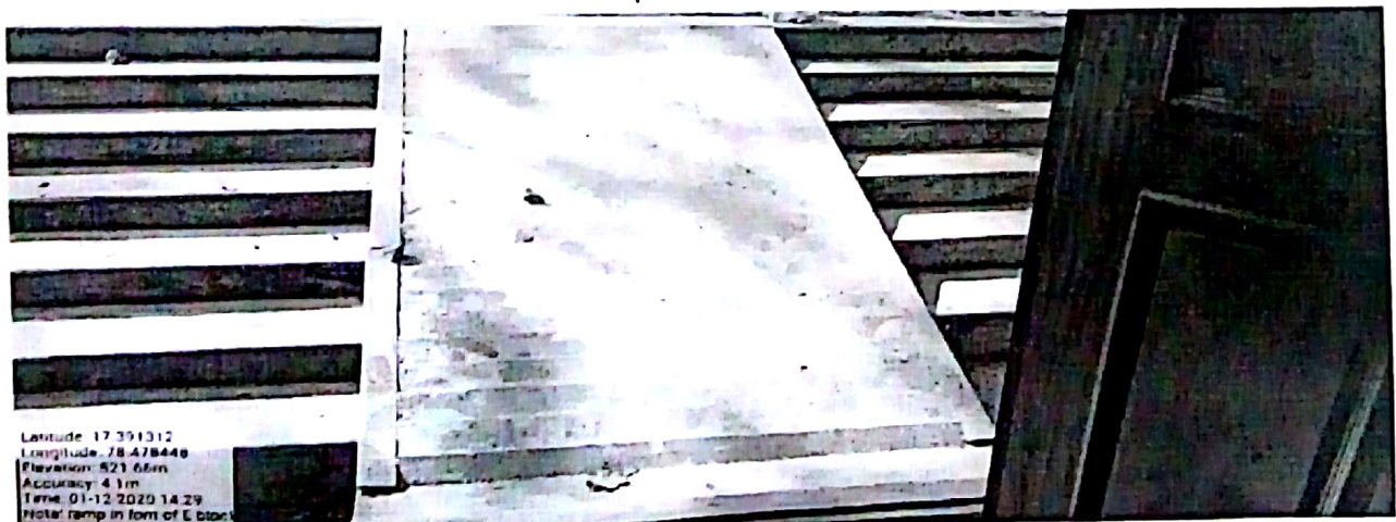
Ramp in E block
