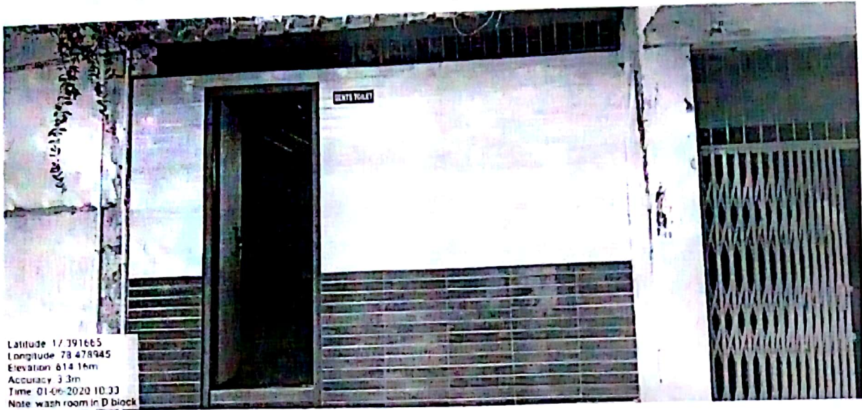
Gents washroom at ground floor near D block
